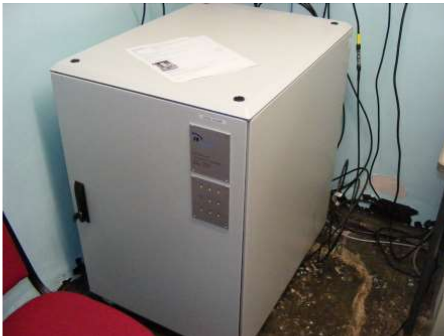
The temperature controlled cabinet that contains the hydrogen maser
